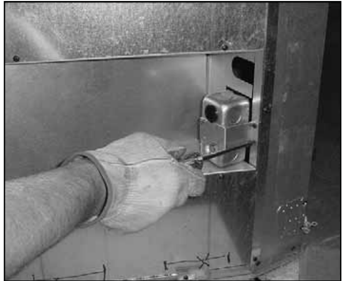
Figure 13.2 Remove Two Screws From Bracket
